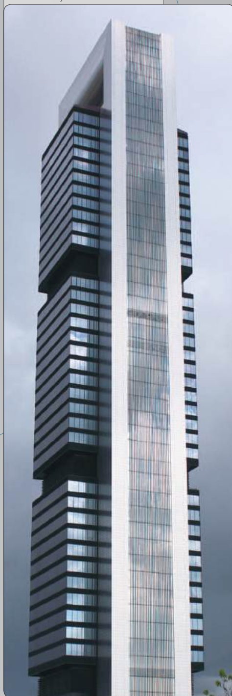
Madrid - Caja Tower
